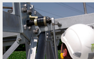
alkitronic ® M operating on electricity pylons. Accurate tightening via torque wrench.
